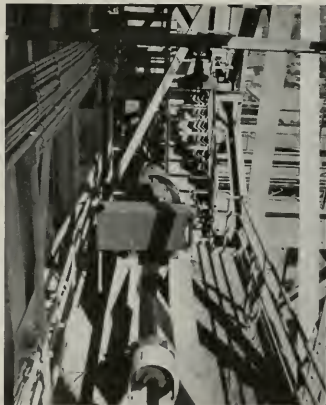
Far right: One of the 8 G. E. 50 hp induction motors which provide motiva power to the bridges. Below is an AK and the forward part of a U. S. cruiser.
